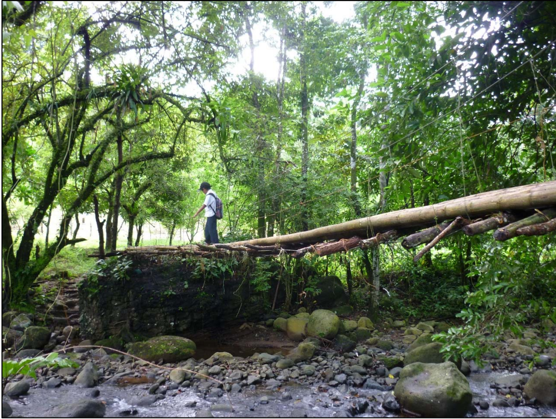
Figure 1: Current Suspension Bridge
